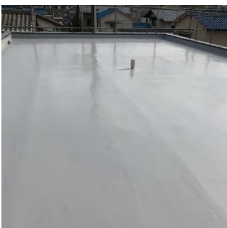
↑屋上防水工事
